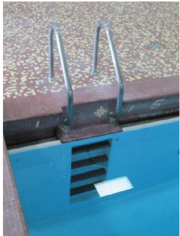
Image 33: Deep End Grab Rails and Recessed Steps
