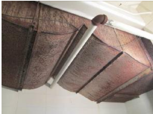
Image 102: Corrosion in Chemical Storage Area
