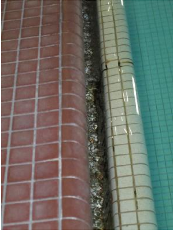
Image 23: 2" Gutter Lip Handhold
