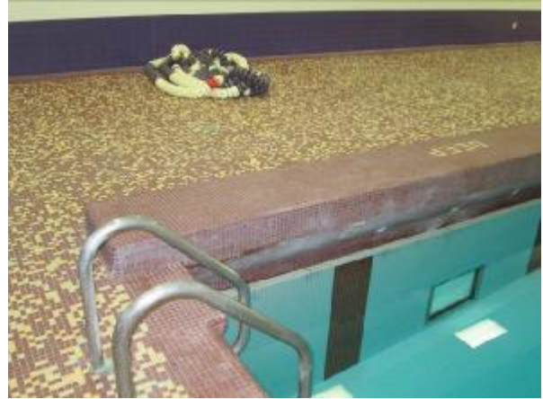
Image 24: Deep End Wall Parapet
