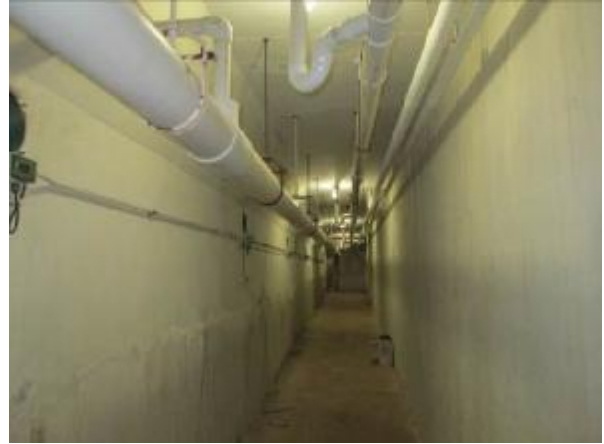
Image 69: Sch 40 PVC Gutter Piping at Pool Perimeter
