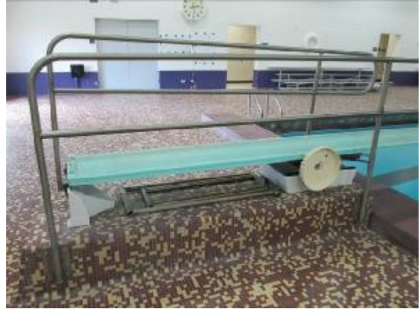
Image 44: Diving Board Stand and Railings
