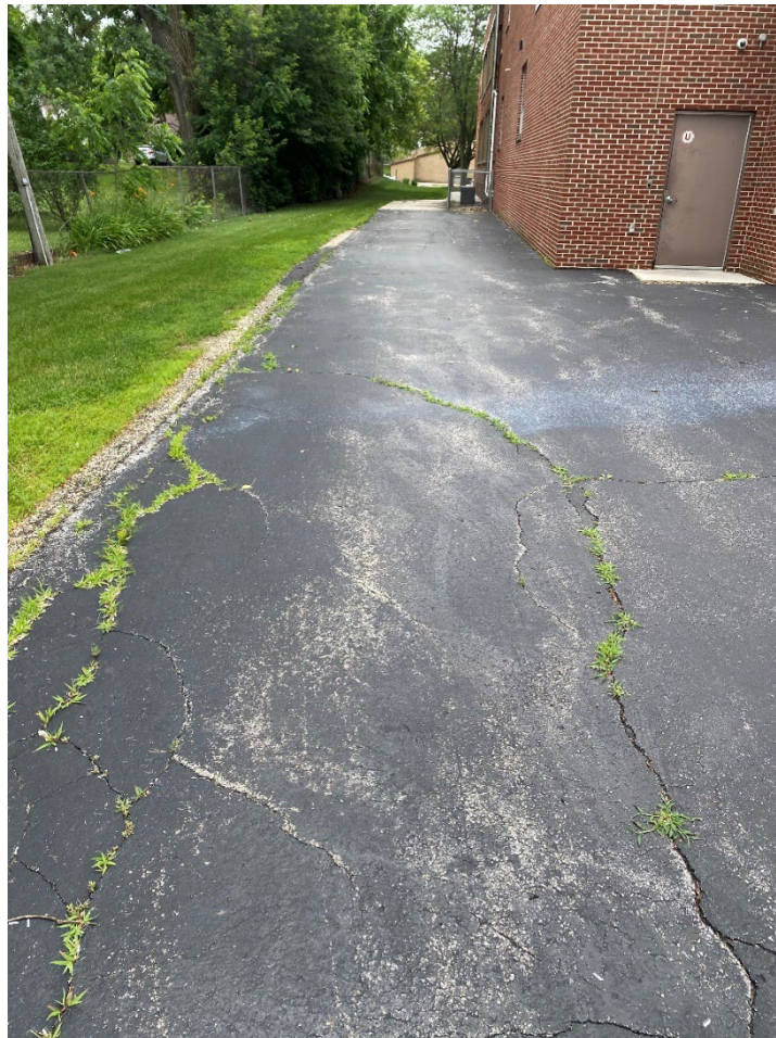
Figure 59: Longitudinal, transverse and block cracking in asphalt on east side of school.
