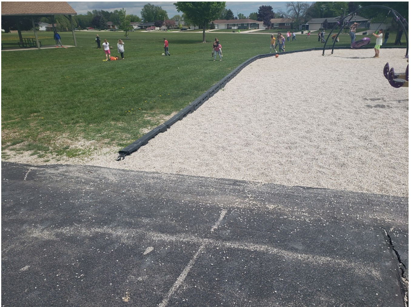
Figure 22: Gravel play area in good condition
