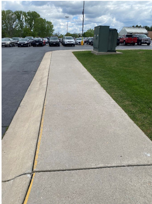
Figure 16: Sidewalk in Student Parking Lot
