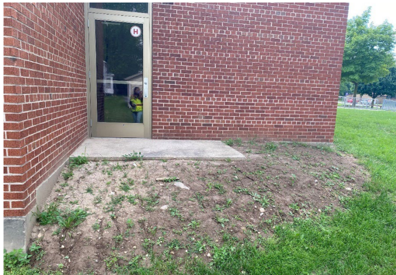
Figure 31: Concrete slab and surrounding grass in good to fair condition on west side of school.
