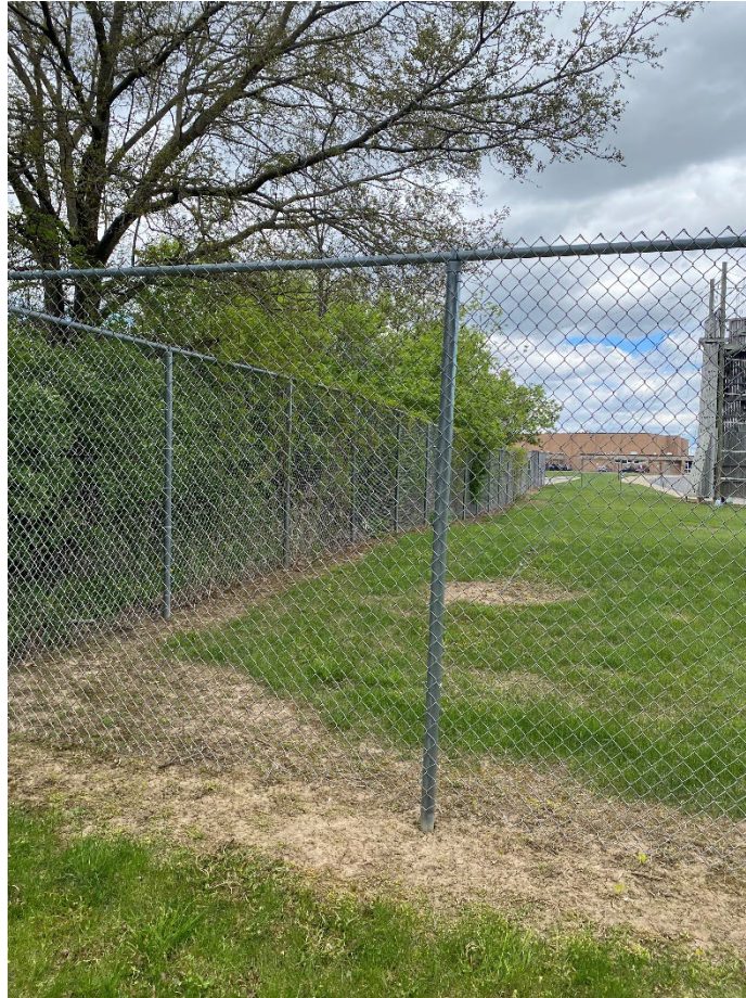
Figure 37: Trees and brush growing into fence on west side of climbing area
