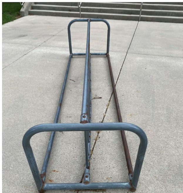
Figure 22: Metal bike racks in fair to poor condition.
