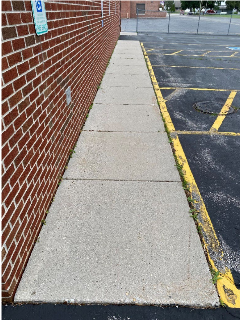
Figure 51: Concrete sidewalk near back east ADA parking stalls in fair condition.
