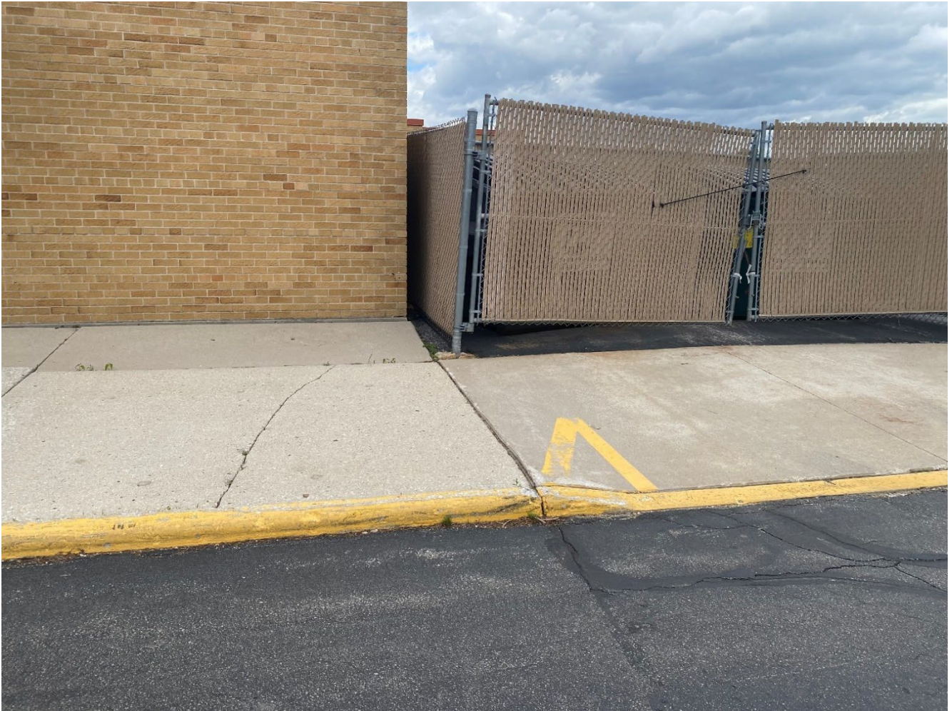
Figure 12: Trash enclosure near north-east corner of south parking lot
