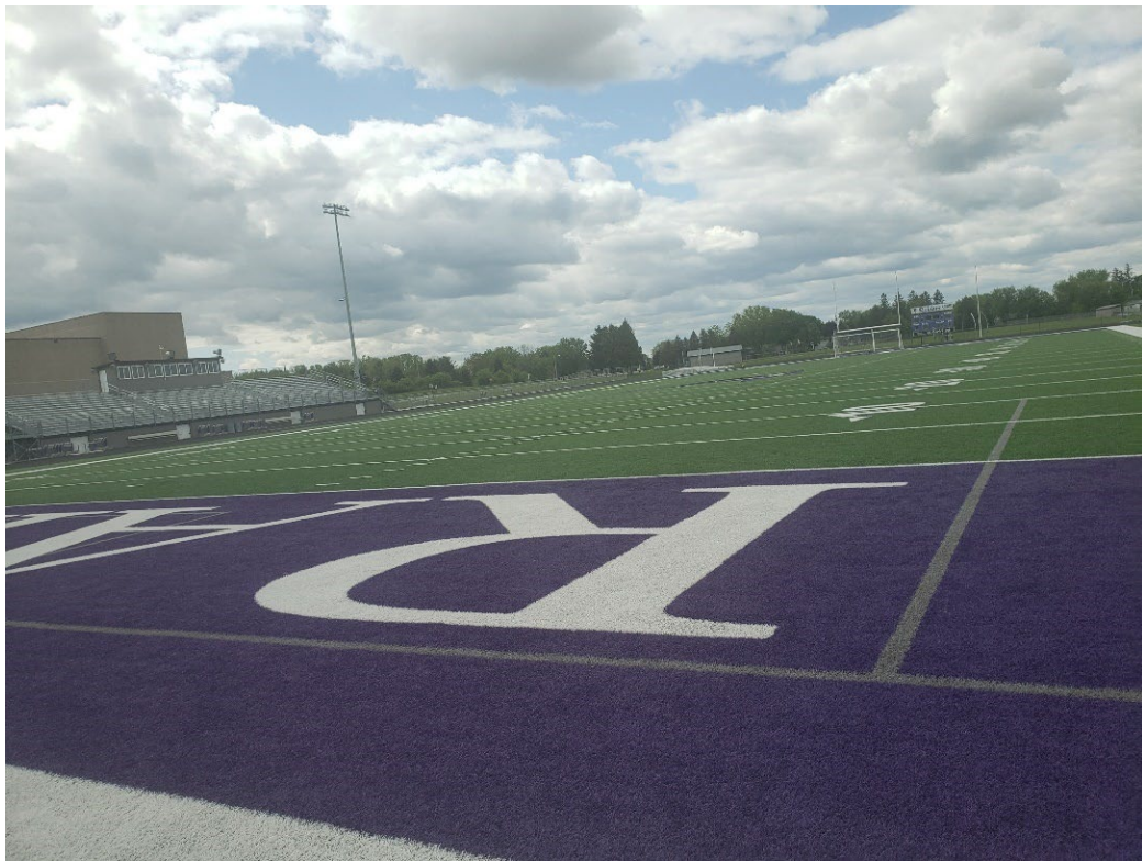
Figure 24: Artificial turf football field in excellent condition.
