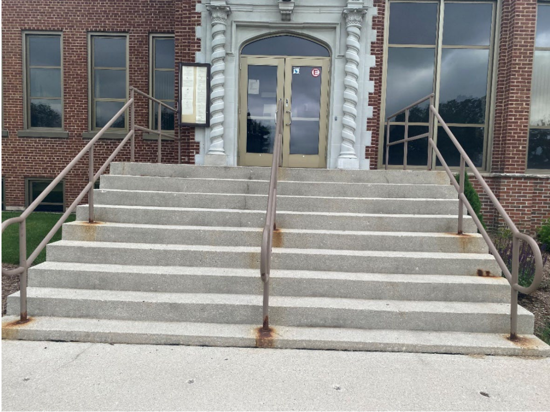
Figure 12: Front center west stairs.
