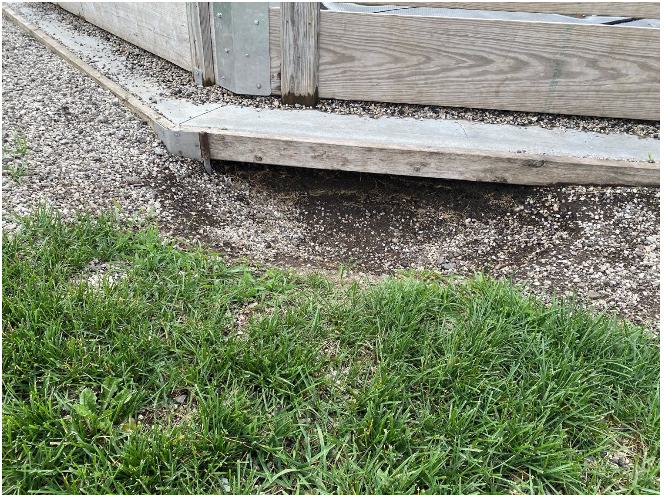
Figure 56: Missing gravel base under wooden octagon play area.
