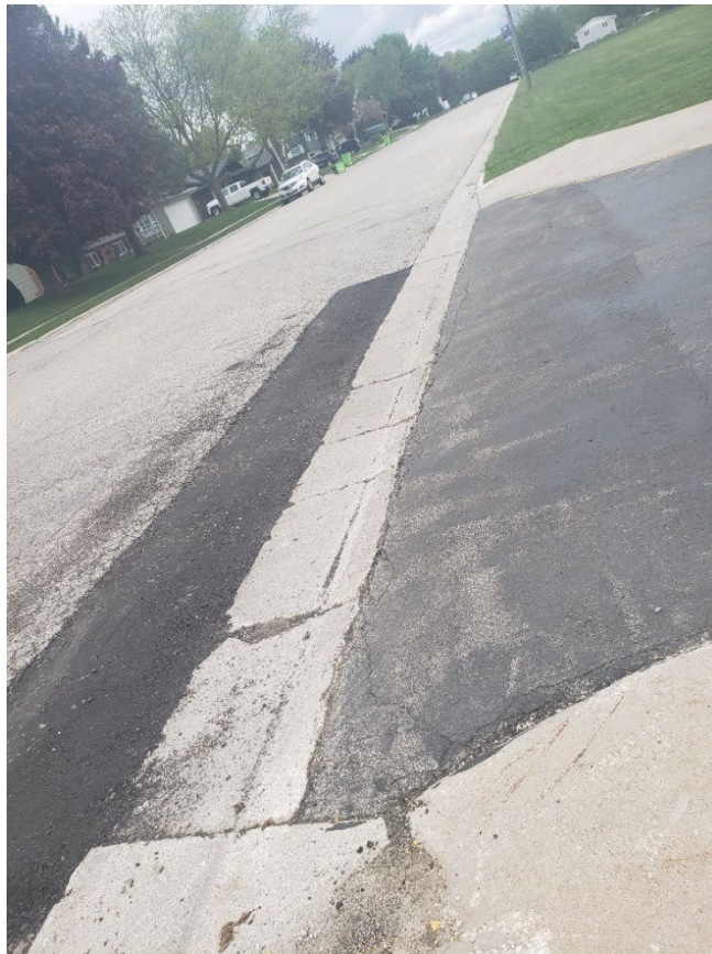
Figure 2: NW Driveway apron in fair condition.
