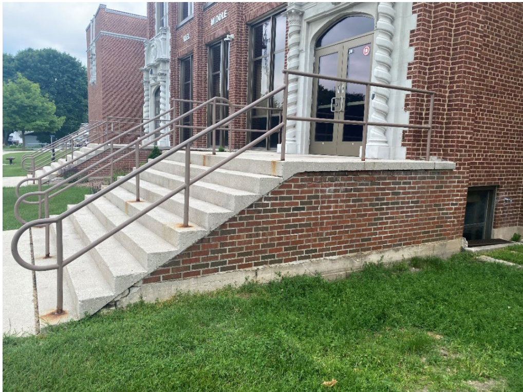
Figure 8: Side of center east concrete stairs.
