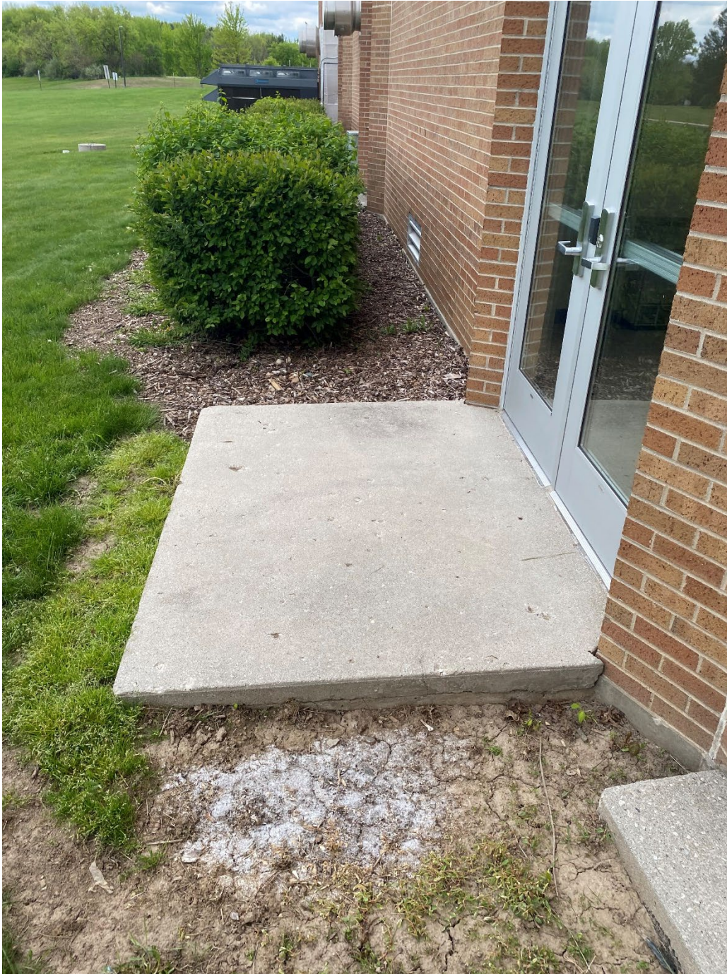
Figure 21: Door landings on east side of building
