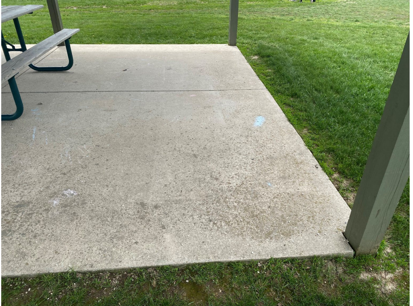
Figure 17: Concrete picnic table pad in good condition
