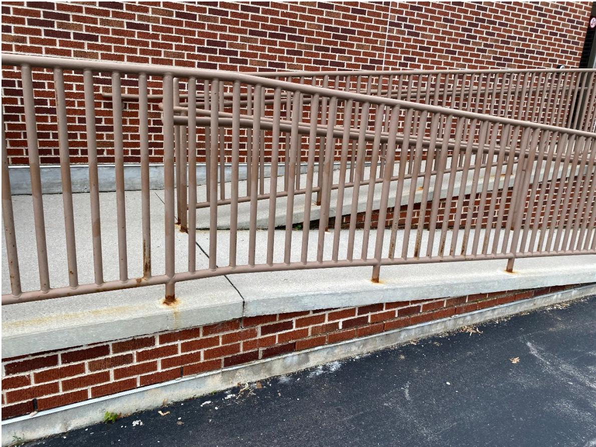
Figure 39: Back concrete ramp in fair condition.
