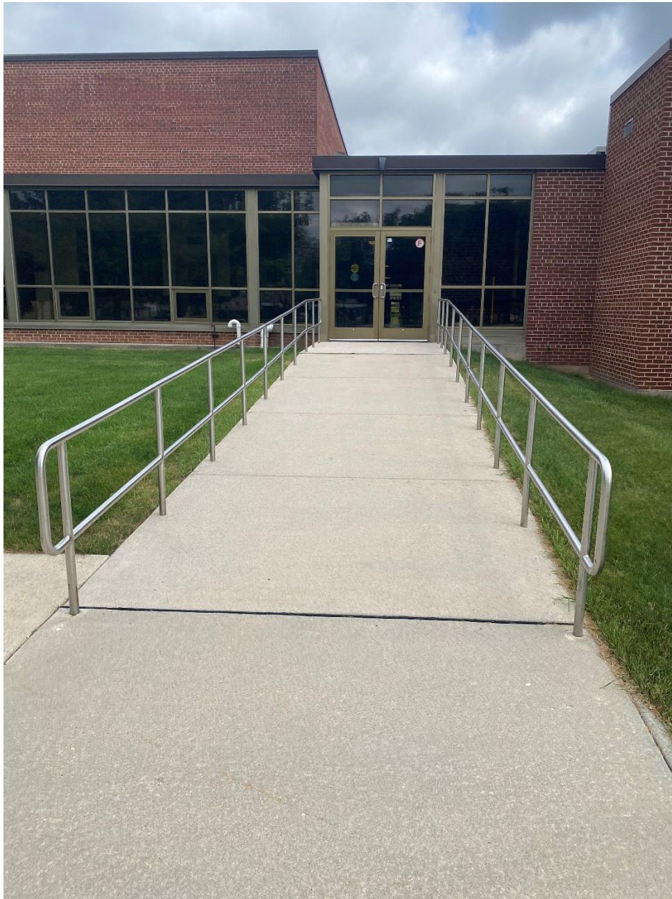
Figure 19: Front concrete ramp in good to fair condition.
