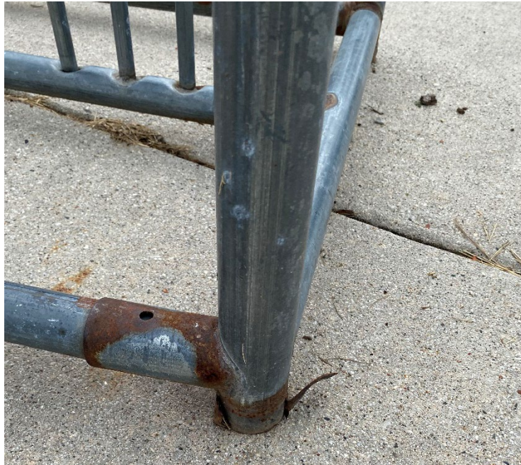
Figure 21: Sharp edges exposed on metal bike rack.
