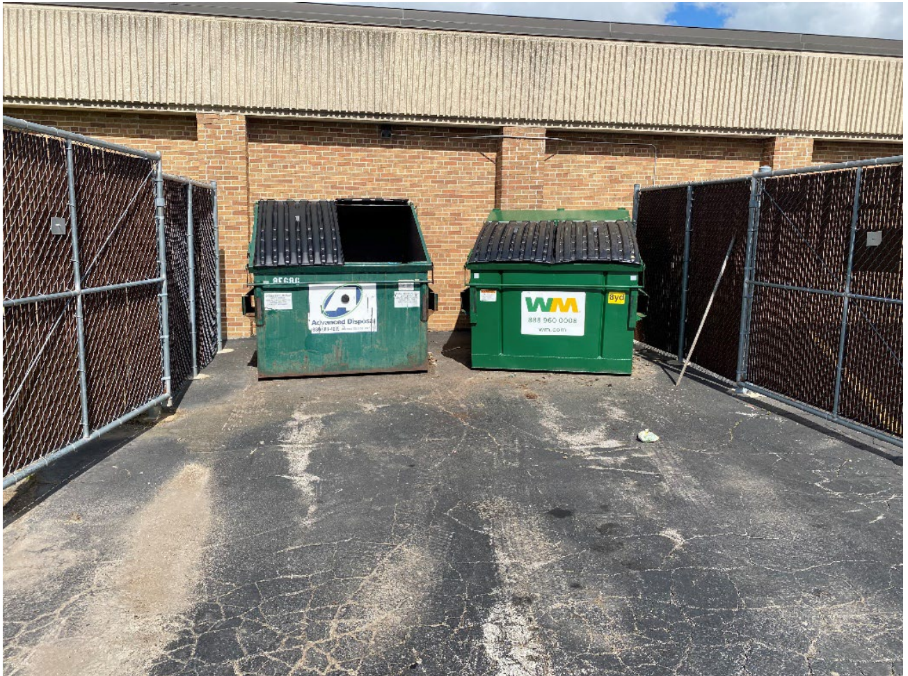
Figure 9: Dumpster enclosure fencing in good condition.
