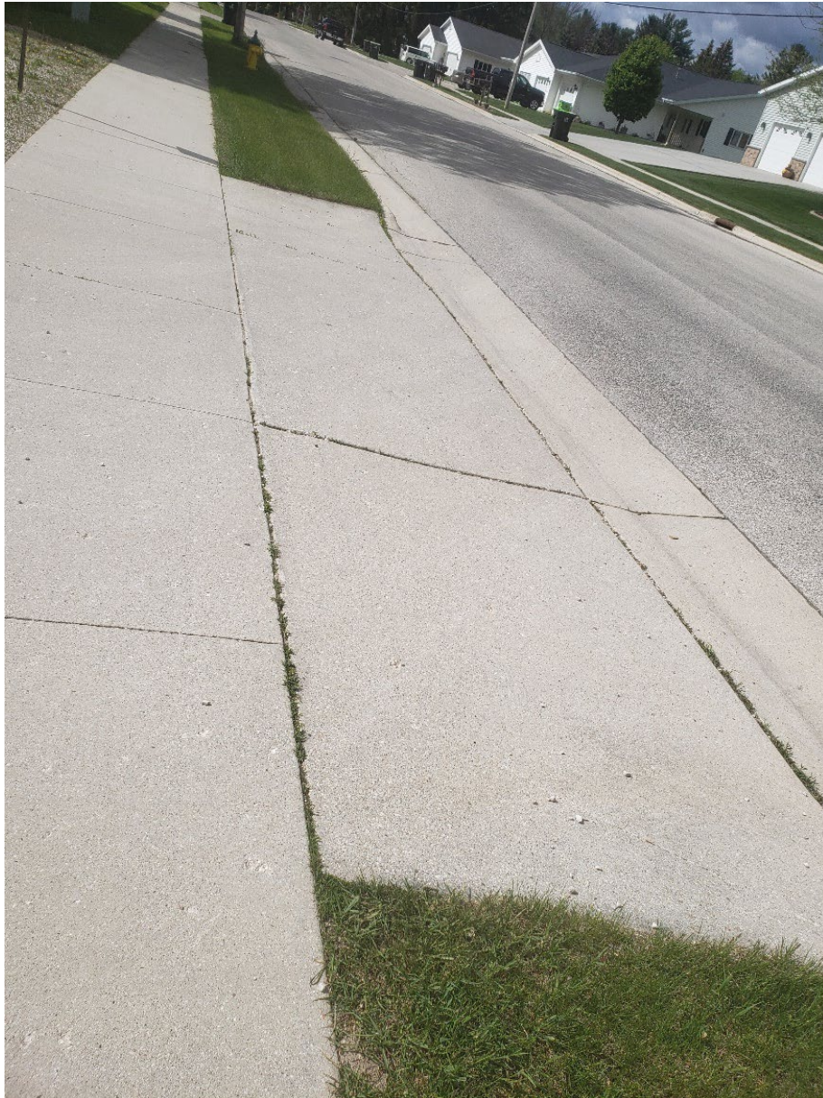
Figure 29: Driveway apron in good condition.
