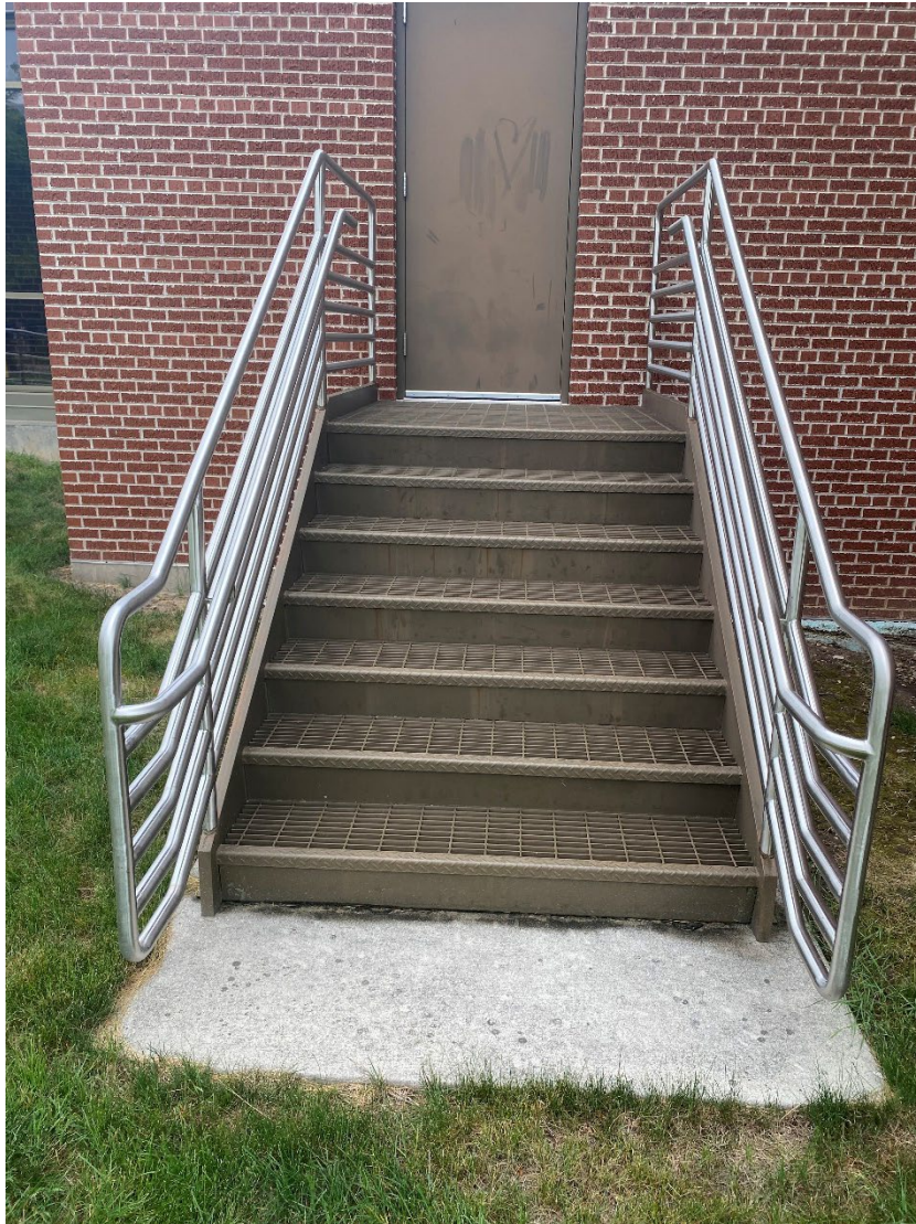
Figure 18: Front metal stair in good condition.
