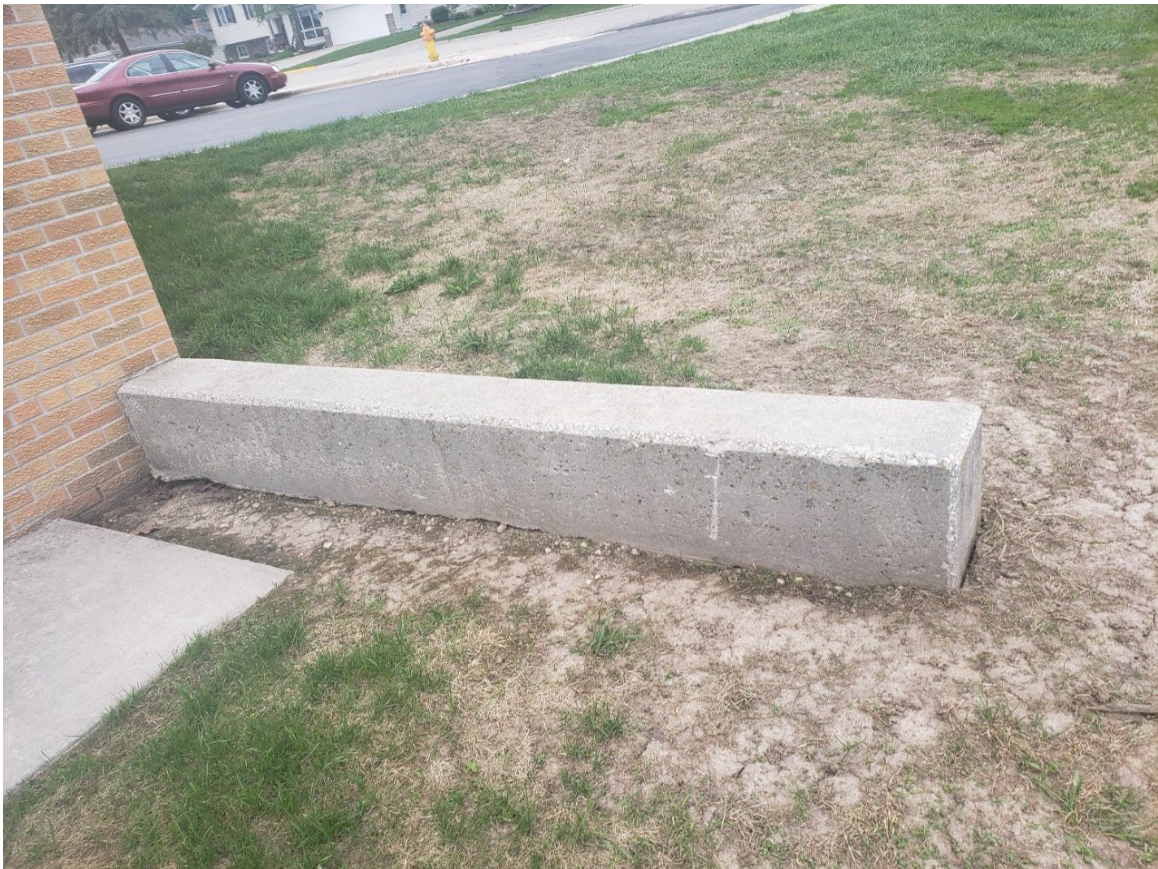
Figure 13: Concrete seating area
