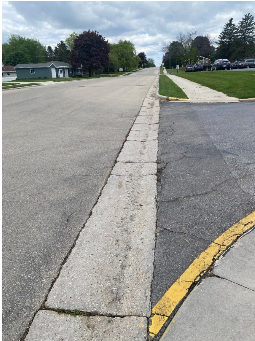
Figure 7: South driveway apron
