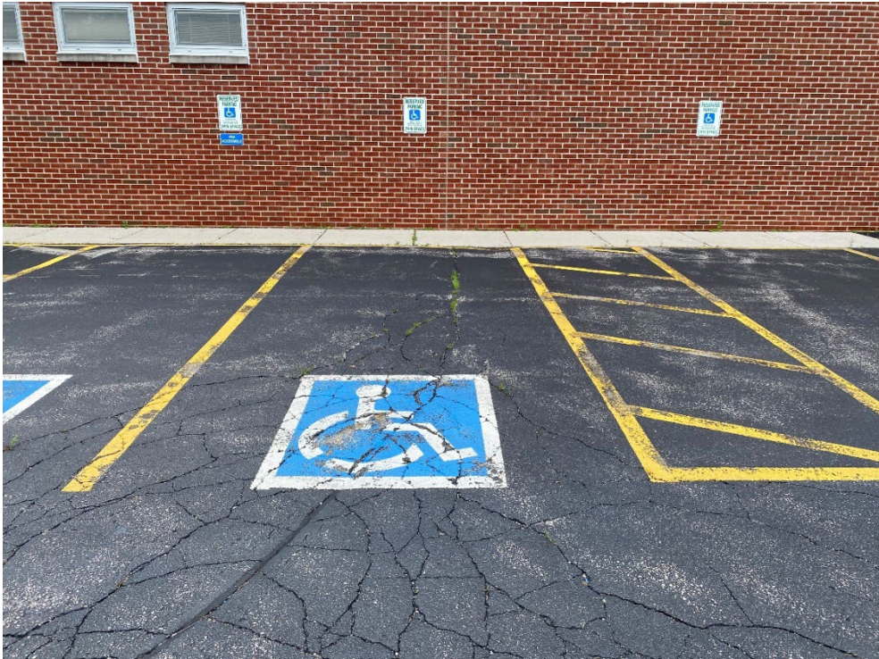
Figure 49: Alligator cracking in ADA stalls on east side of back of school.
