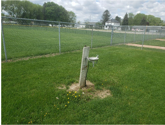
Figure 27: Water fountain in between practice baseball fields in poor condition
