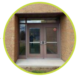
Hollow Metal Doors with Hollow Metal Storefront
