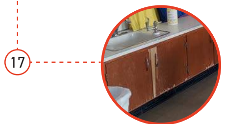
Wood and Laminate Casework
